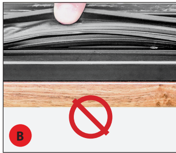
Fig. 12. Pull the side of the gasket to check its installation. A: CORRECT; gasket channel is NOT visible. B: INCORRECT; gasket channel is visible.
