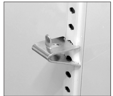
Fig. 4. Installed shelf clip.
