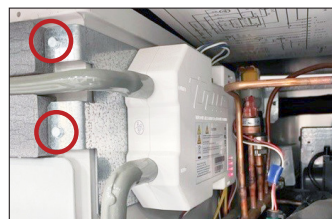
Fig. 3. TRUEZONE UV system side view. TRUEZONE bracket screw locations.
