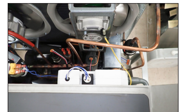
Fig. 2. TRUEZONE UV system top view.
