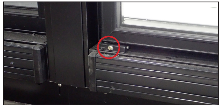
Fig. 4. Door tension adjustment screw location at the bottom of the door.
