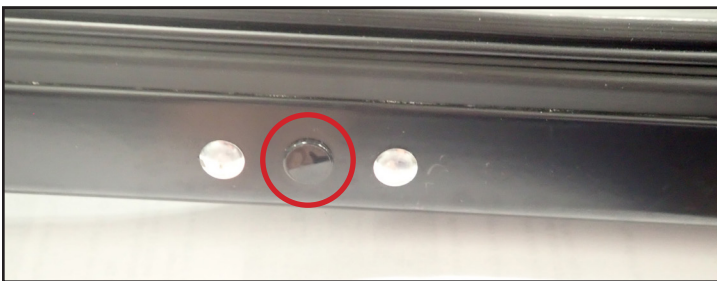
Fig. 15. Plastic cap in the door's bottom.
