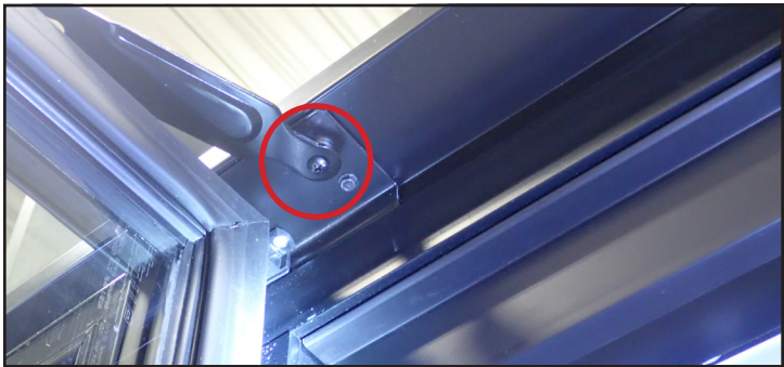
Fig. 9. Hold open bracket screw location at the top of the door.
